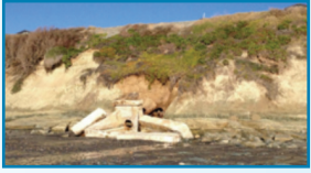
A. Drainage Improvements
