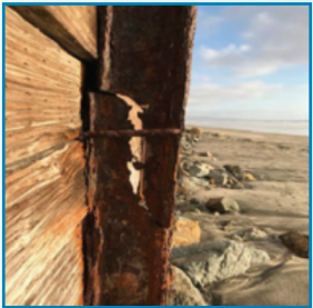
C. Retaining Wall Improvements
