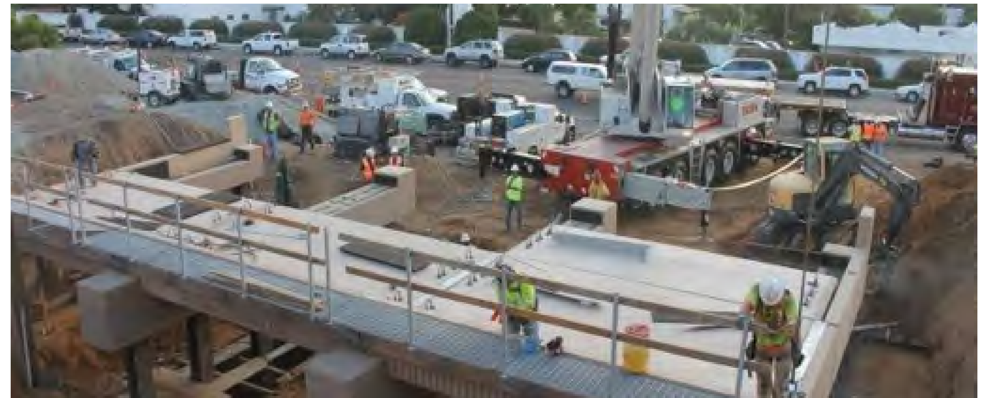
Santa Fe Undercrossing construction images
