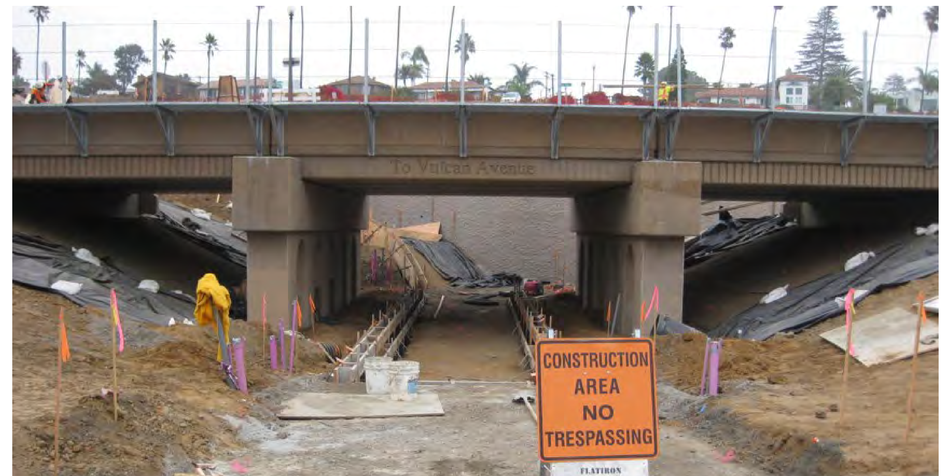
Santa Fe Drive Undercrossing construction which opened in 2013
