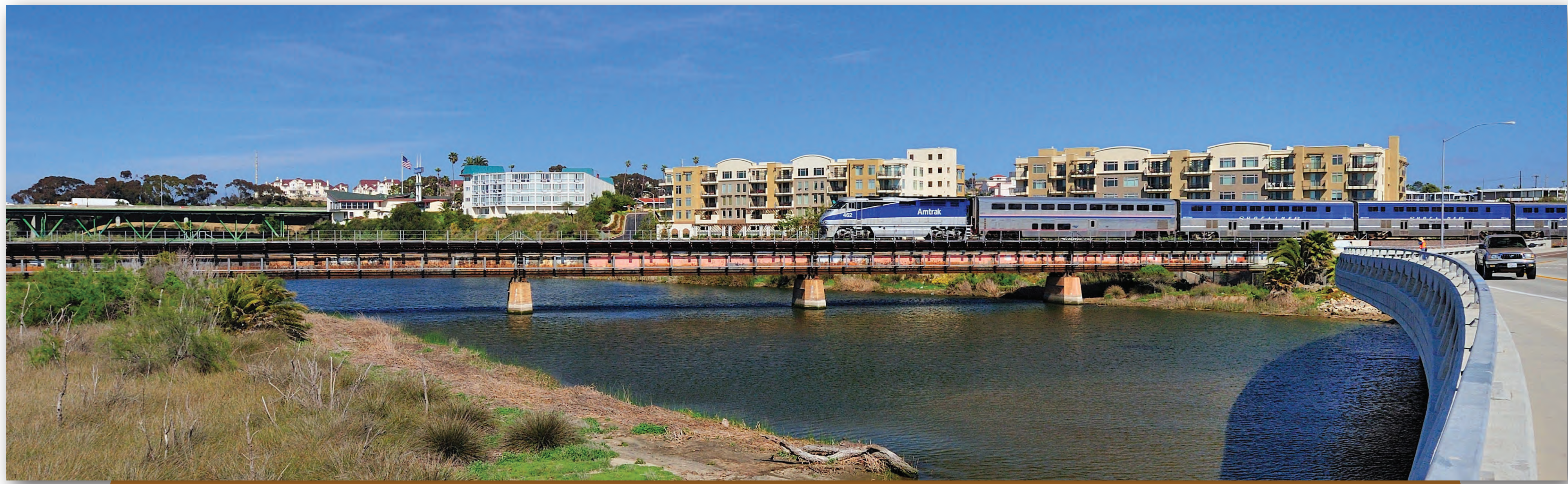
San Luis Rey River Rail Bridge
