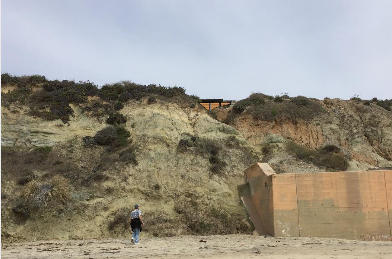
CIDH piles and lagging wall to support access road
