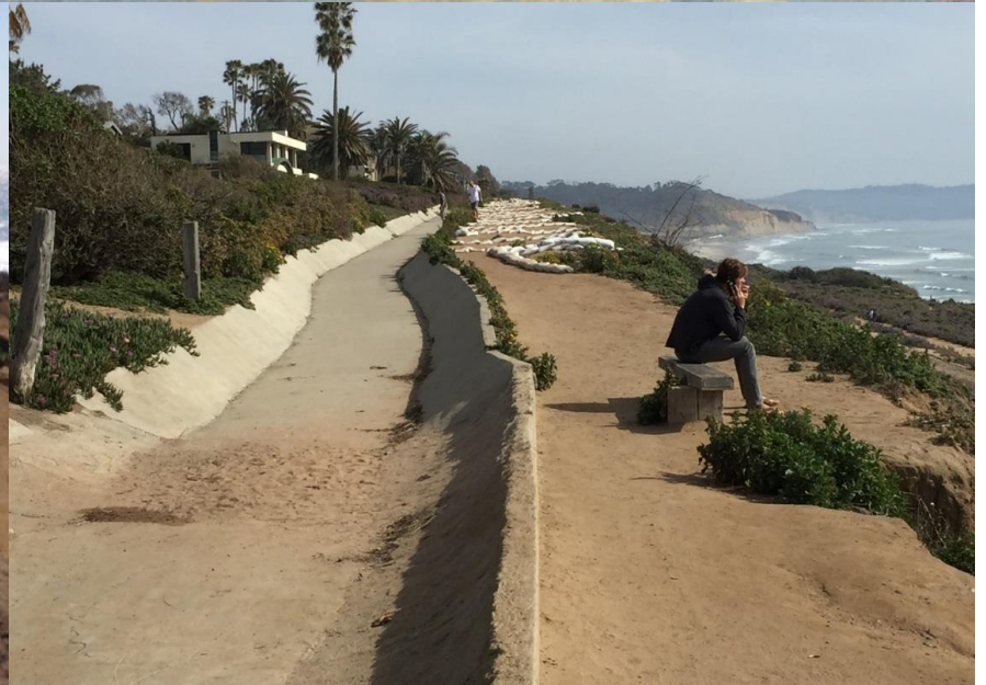
New concrete drainage channel to replace existing structure
