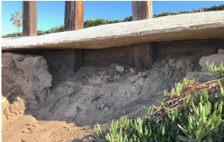
CIDH piles and lagging wall to support drainage channel
