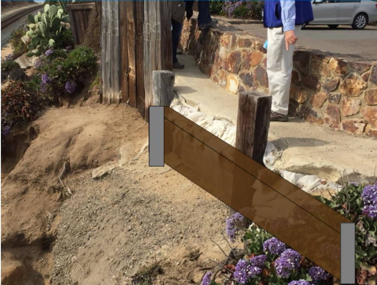
Timber posts and lagging to repair flood wall
