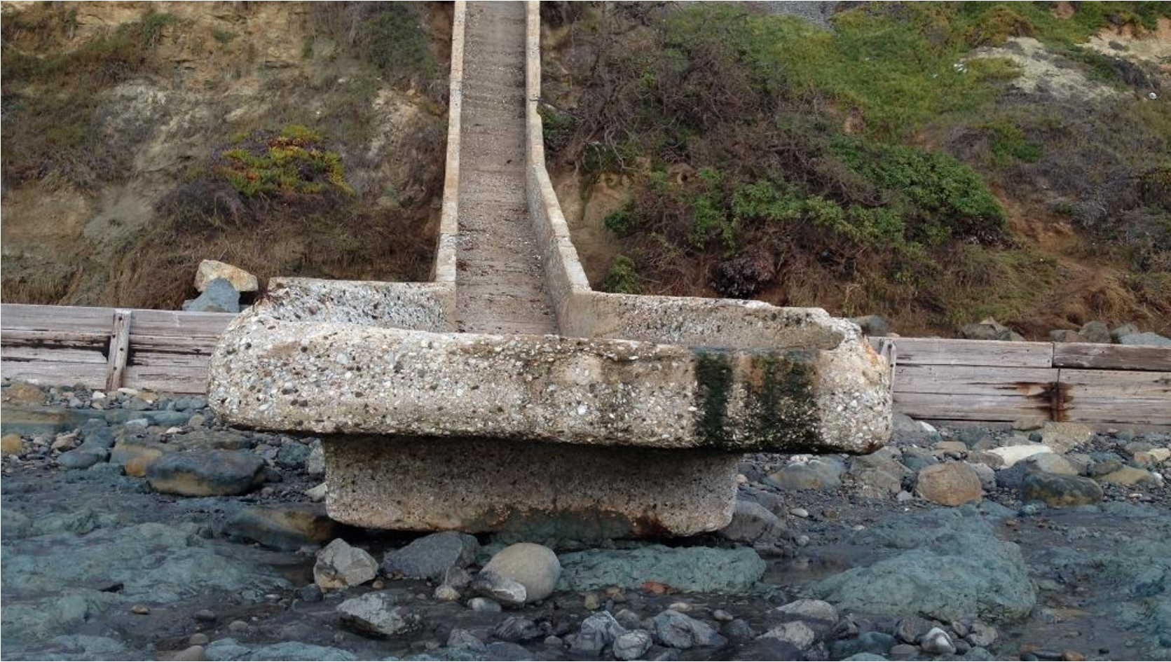
Stabilize outfall with concrete
