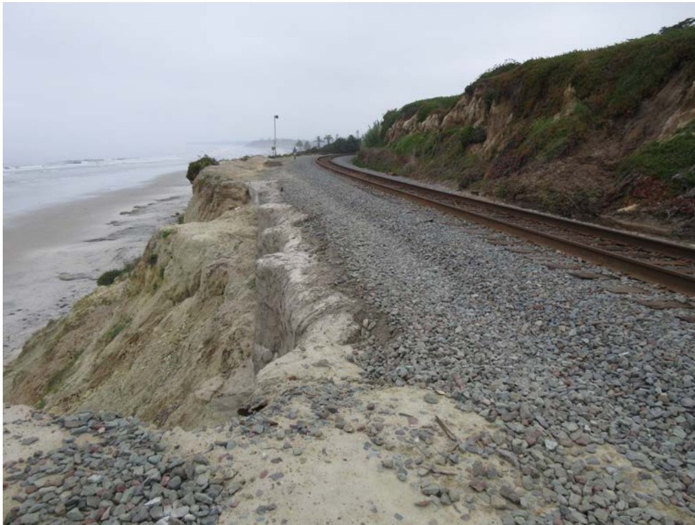
Photo 1. Looking north at eroded, unvegetated bluff adjacent to railroad in the northern part of the study area.
