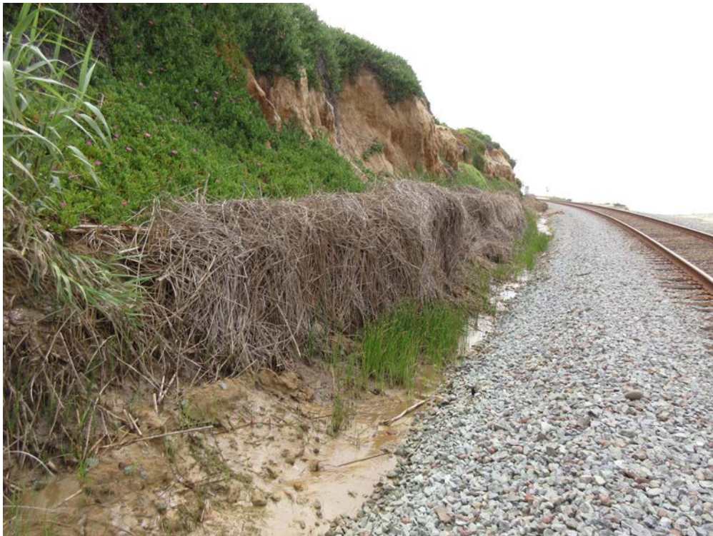
Photo 2. Looking south at freshwater marsh within an upland-constructed swale adjacent to the railroad in the northern part of the study area.
