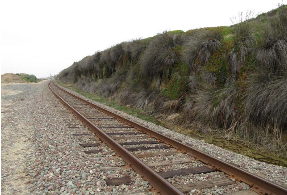
Photo 9. Looking north at the railroad in the southern part of the study area. Cismontane alkali marsh is present on the bluff face east of the railroad where seepage from irrigation and urban runoff provides a source of hydrology. Disturbed freshwater marsh occurs in the upland-constructed swale at the base of the bluff, paralleling the railroad.
