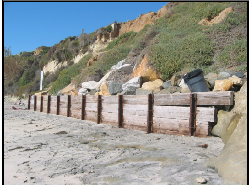
Figure 8. Timber Wall at Station 1514
