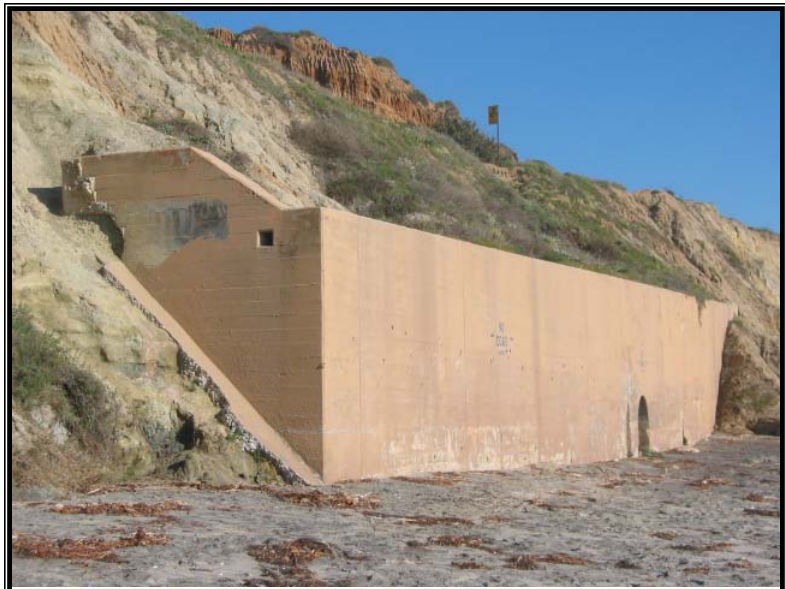
Figure 2. Gravity Wall at Anderson Canyon (BR 245.4)
