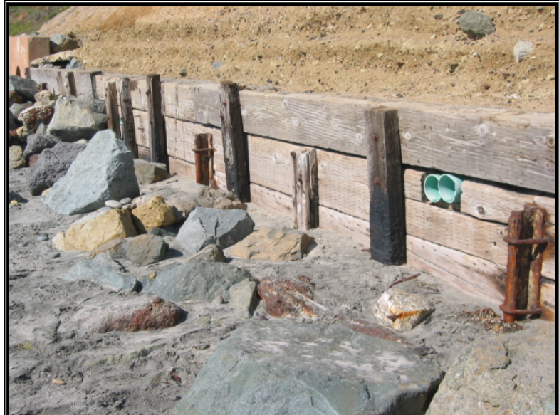
Figure 9. Timber Wall at Twelfth Street
