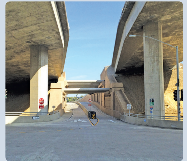
Existing north-facing Direct Access Ramp
