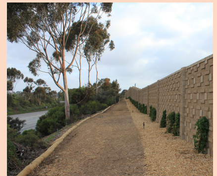
A typical sound wall design along I-805. Designs for the sound walls will vary by location and may include masonry, glass, or other materials.
