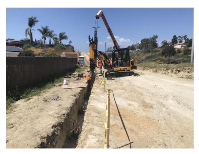
This photo demonstrates how close homes are located next to the highway. Here the cast and drill holes have been prepared and a concrete foundation will soon be installed. Nearly 70 percent of the sound walls have been erected.
