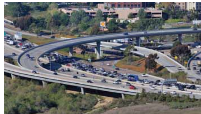
The I-5/SR 56 Interchange Project will reduce traffic congestion for both the highway and surface streets in area.
