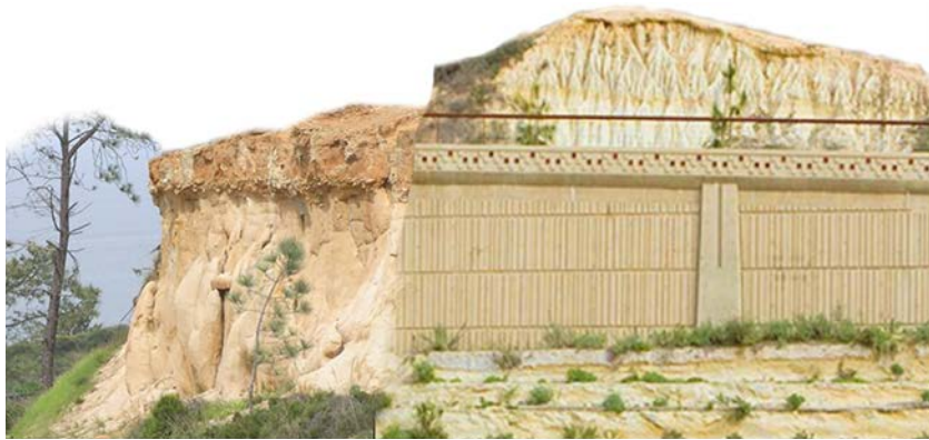
In Solana Beach, the rational character of the surrounding bluffs was the basis for the design of the walls
