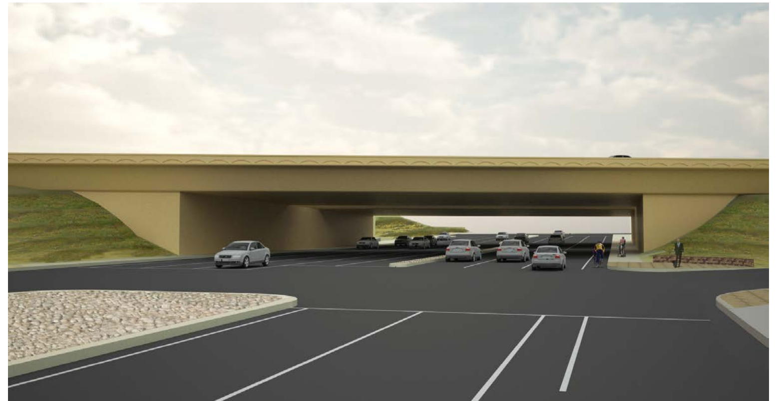
View of one-span undercrossing from approach
