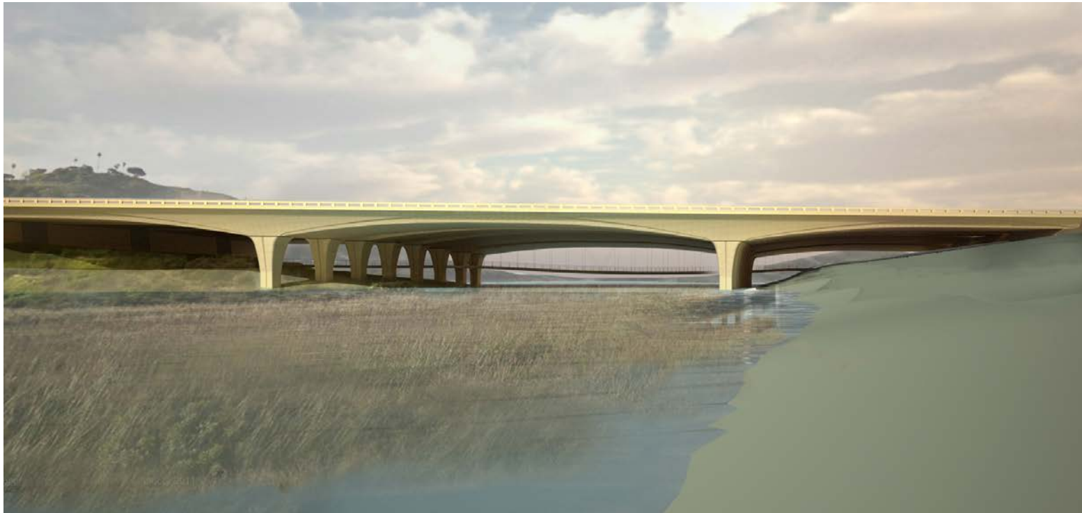
View of lagoon bridges at lagoon edge
