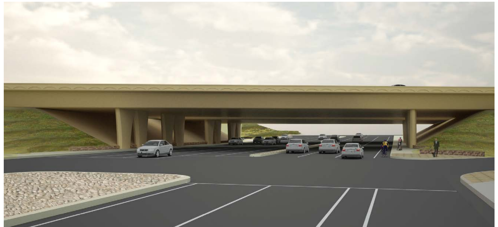
View of gateway from approach with columns at back of sidewalk
