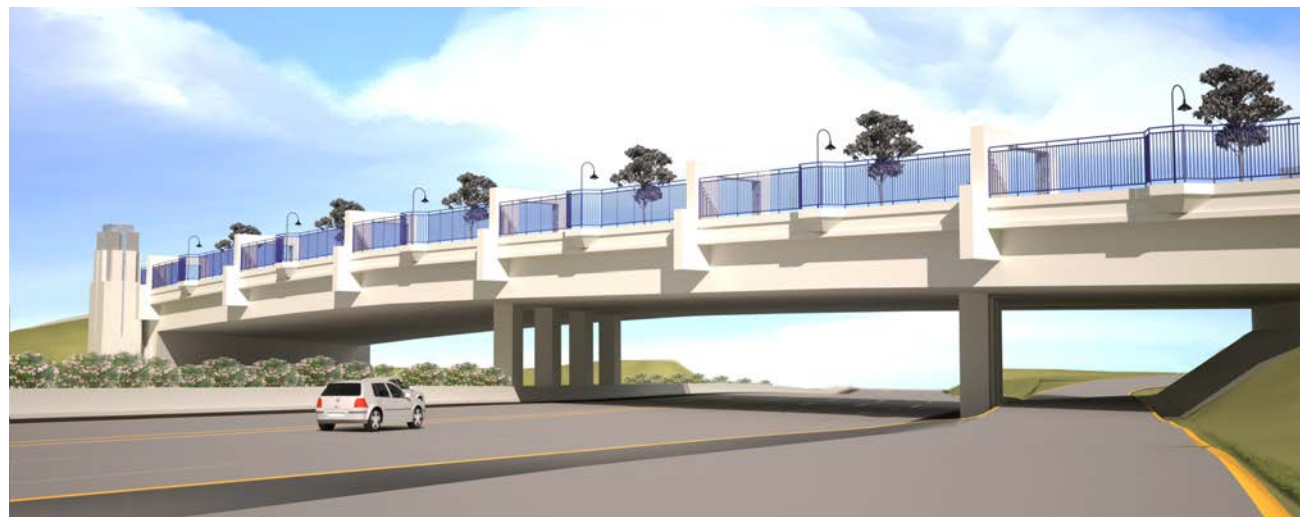
The gateway overcrossing features a processional arch along the pedestrian path and is anchored by four monumental structures at the edges on each side
