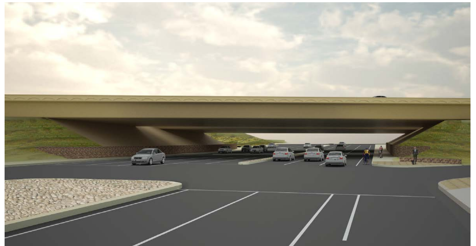
View of one-span undercrossing from approach
