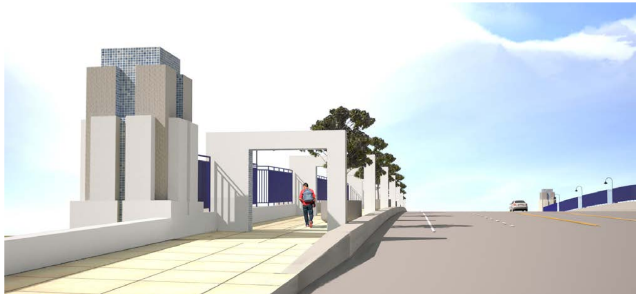
View of the monument's composition, including ceramic tiles, vertical formliner texture, and sandblasted concrete
