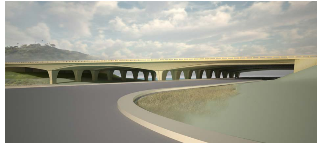
View of lagoon bridge looking south-west
