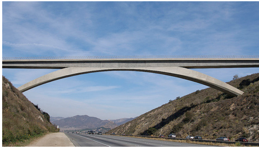
The West Lilac Road Bridge over Interstate 15
