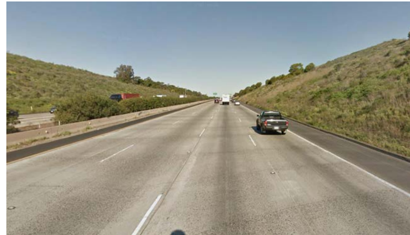
The visual impact of tall manufactured slopes can be mitigated by plant material
