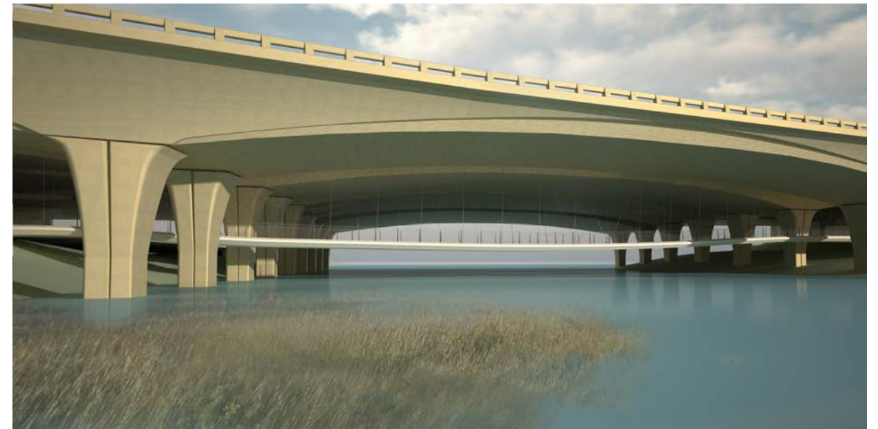
Pedestrian bridge suspended from main structure
