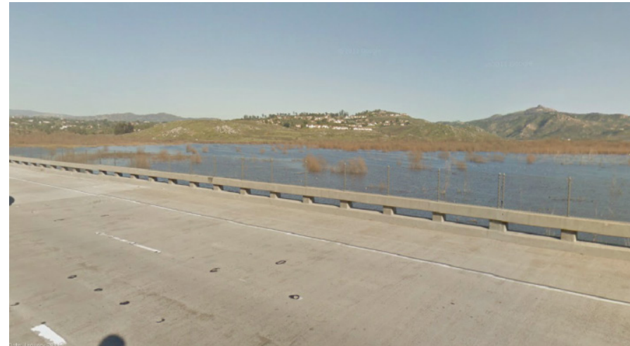
An example of a barrier maintaining an open view over Lake Hodges
