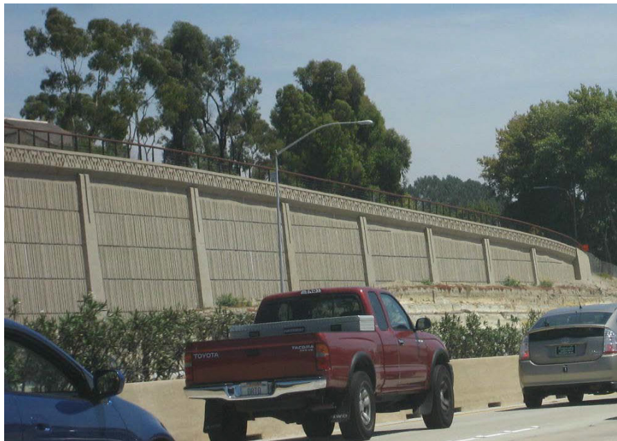
The Lomas Santa Fe interchange retaining walls in Solana Beach
