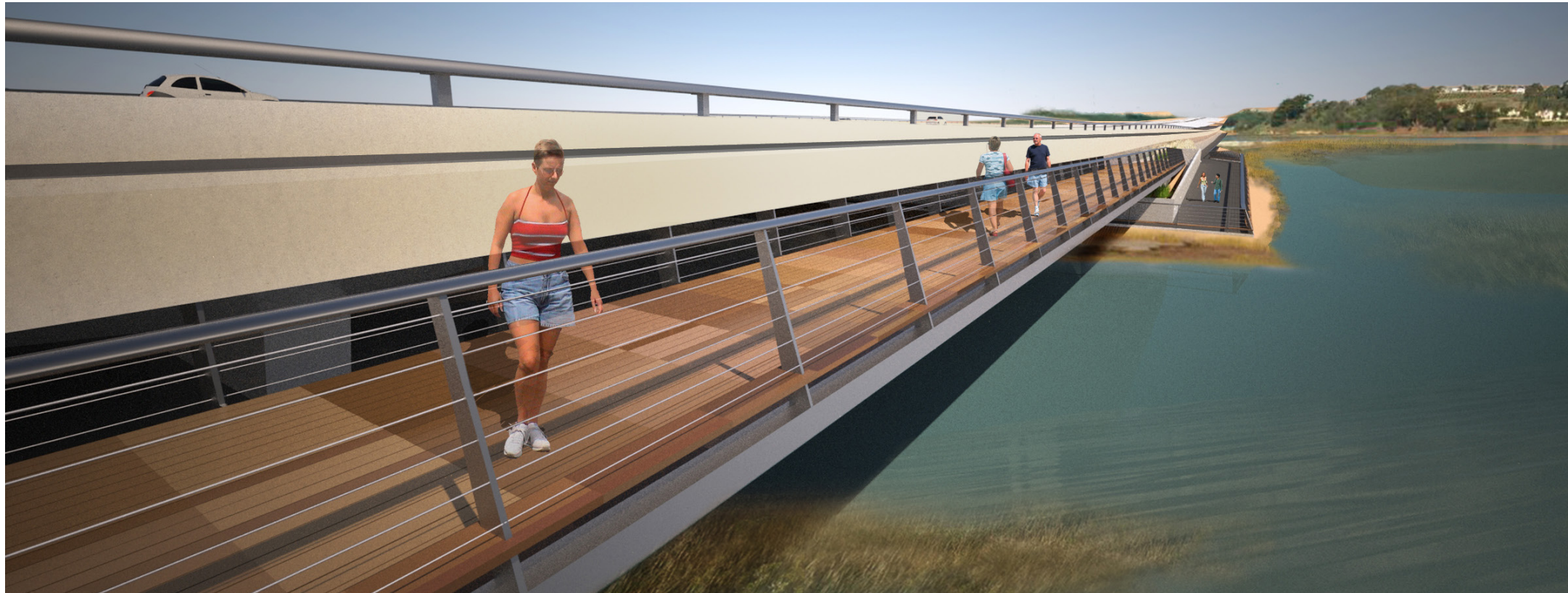
View of the pedestrian walkway adjacent to the lagoon bridge.
