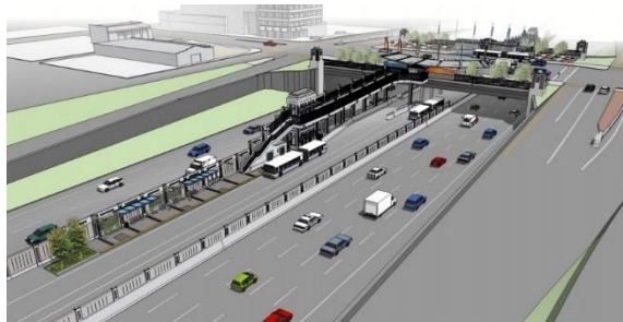
Proposed station at University Avenue, looking north. Platform to be connected with street-level plaza and bus stops using stairs, elevator and pedestrian bridge.
