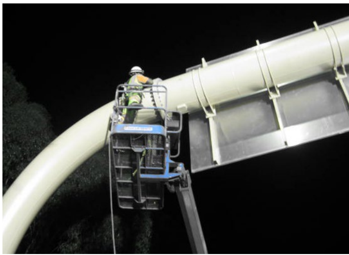
Construction crews install overhead sign structures over SR 15.
