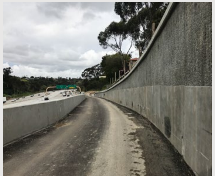
The SR 15 Commuter Bikeway looking north from Adams Avenue: progress on the concrete barrier that separates the bikeway from the freeway, the paved path, and the retaining wall that will align the path.
