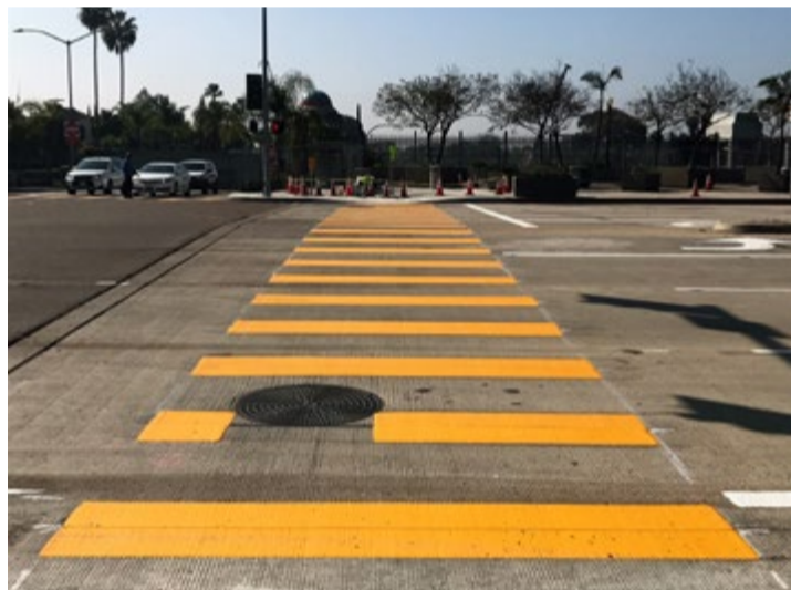
Upgraded crosswalk on El Cajon Boulevard at SR 15.
