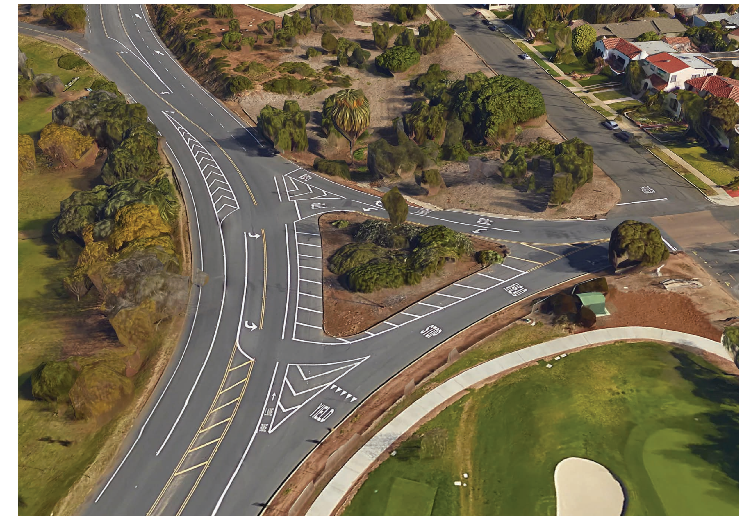
There is currently no safe crossing option from 28th Street to Florida Drive within Balboa Park. Introducing a roundabout to this intersection will enhance safety and connectivity.
