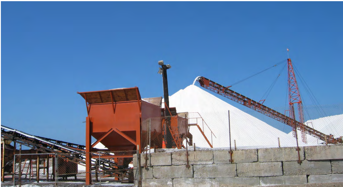
View of salt processing at South Bay Salt Works from Bay Boulevard
