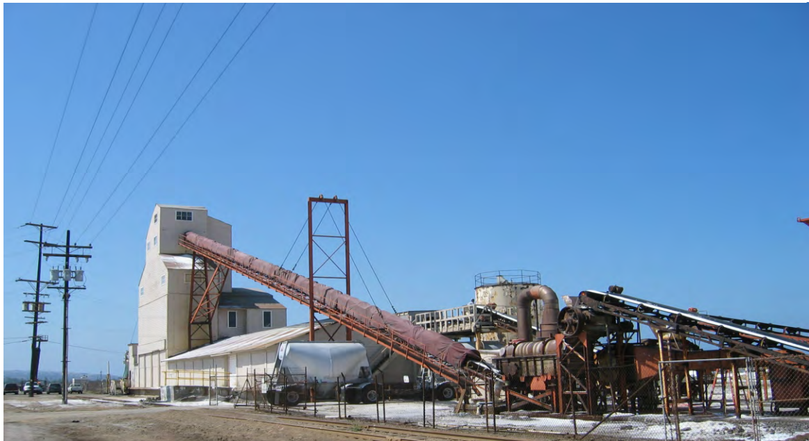
View of South Bay Salt Works main facility looking southwest from Bay Boulevard
