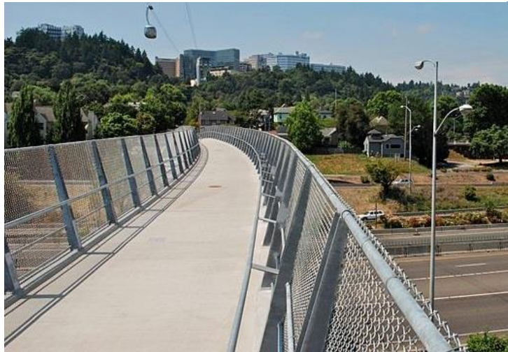
Figure 6.1 Class I Bikeway/Multi-Use Path on Bridge
