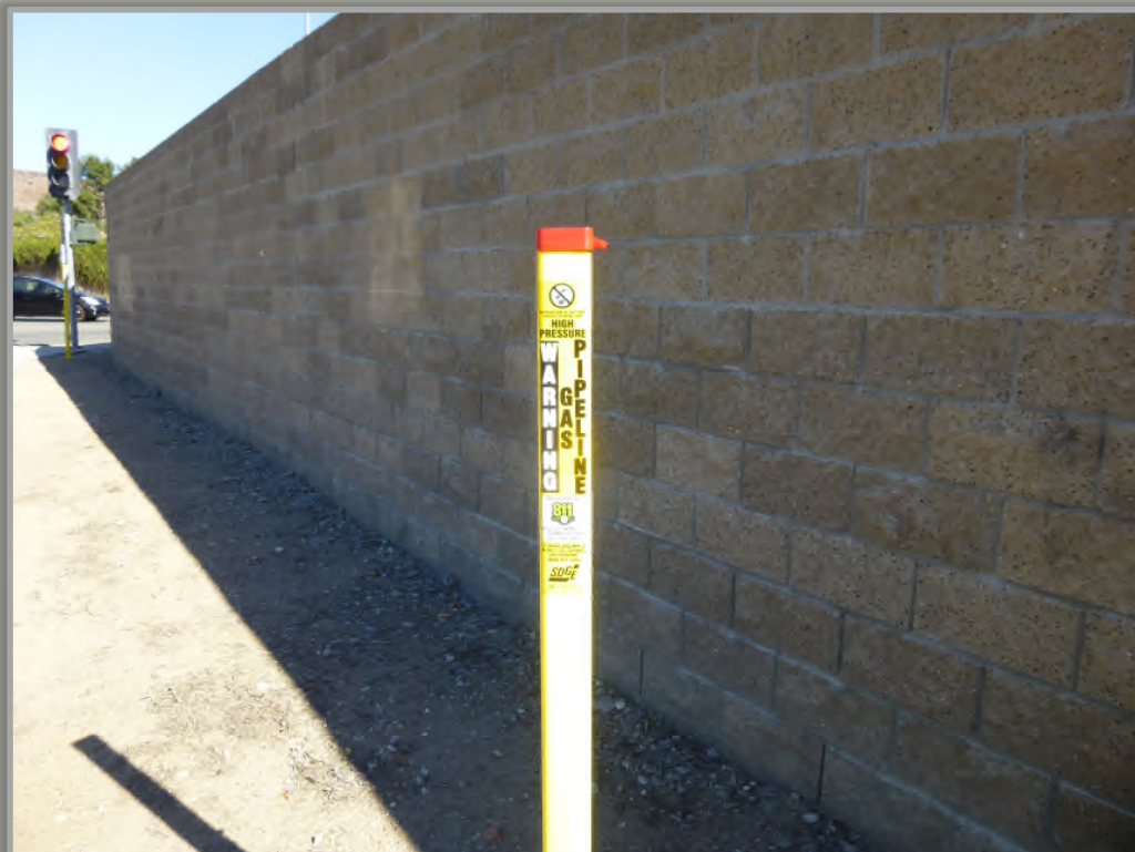
Photograph 6: Viewing north at sign indicating a 24" high pressure gas line is present underground. This line extends along eastern shoulder of West Hills Pkwy near the starting point of the Option 2 bikeway entrance. Unless extensive excavation will take place, it is unlikely this gas line will be disturbed.
