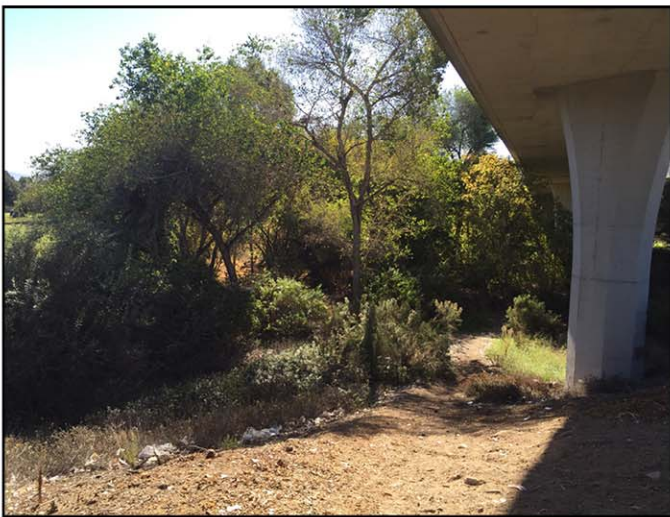
Photograph 5: SR-52 over San Diego River near the southwest corner of the project site.
