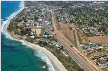
Aerial View of Project Corridor
