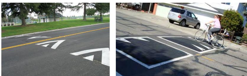
Speed cushions are vertical deflections in the road that encourage people driving to slow. They include wheel cutouts to allow larger vehicles like emergency vehicles and small vehicles like bicycles to pass through easily. Speed cushions are typical speed and volume treatments for Bike Boulevards.
