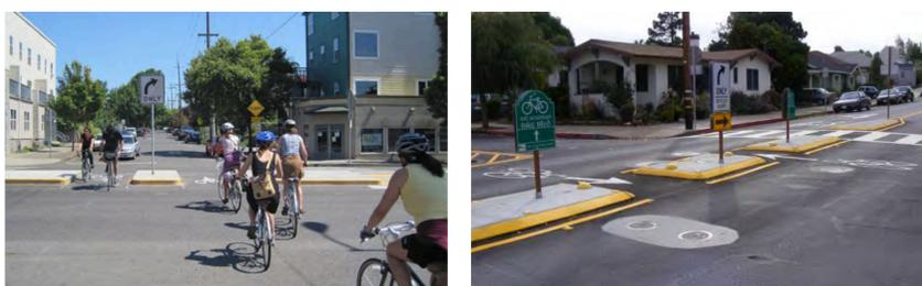
Median island traffic diverters require drivers to turn left or right, rather than driving through an intersection, while allowing people walking and biking to travel through the intersection. They are designed to reduce cut-through traffic and create a safer and more comfortable experience for people biking and walking by lowering traffic volumes and speeds.
