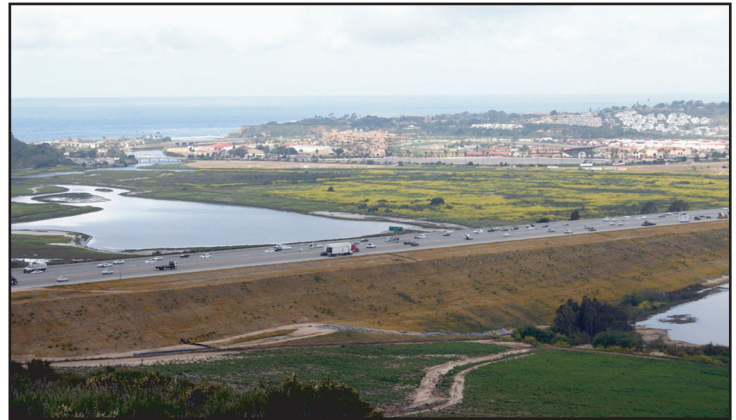
The I-5 freeway leads motorists through diverse land use areas and sensitive habitats. The Del Mar Fairgrounds, dense residential neighborhoods and the San Dieguito Lagoon can all be seen from the freeway.
