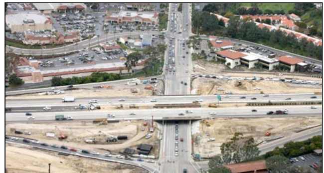
Lomas Santa Fe and I-5 Interchange looking west.
