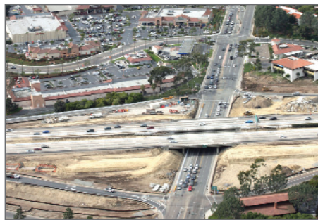
Recent construction activity
