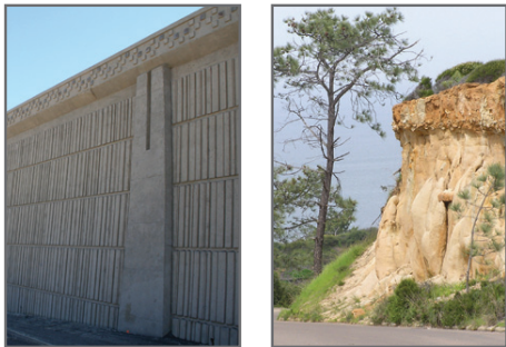
New retaining walls reference surrounding landscape
