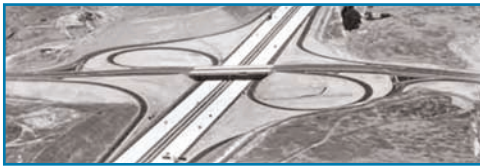
View of La Jolla Village Drive and I-5 when first built fifty years ago.
