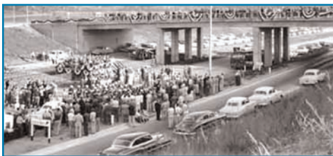
Photo of the I-5 ground-breaking held in 1957 at the Vista Way Bridge, currently known as SR 78.
