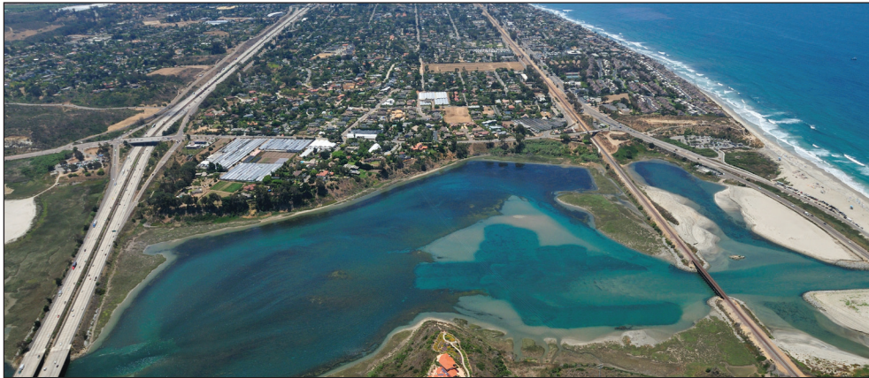
The I-5 and LOSSAN rail line in North County traverses through scenic and unique natural environments.
