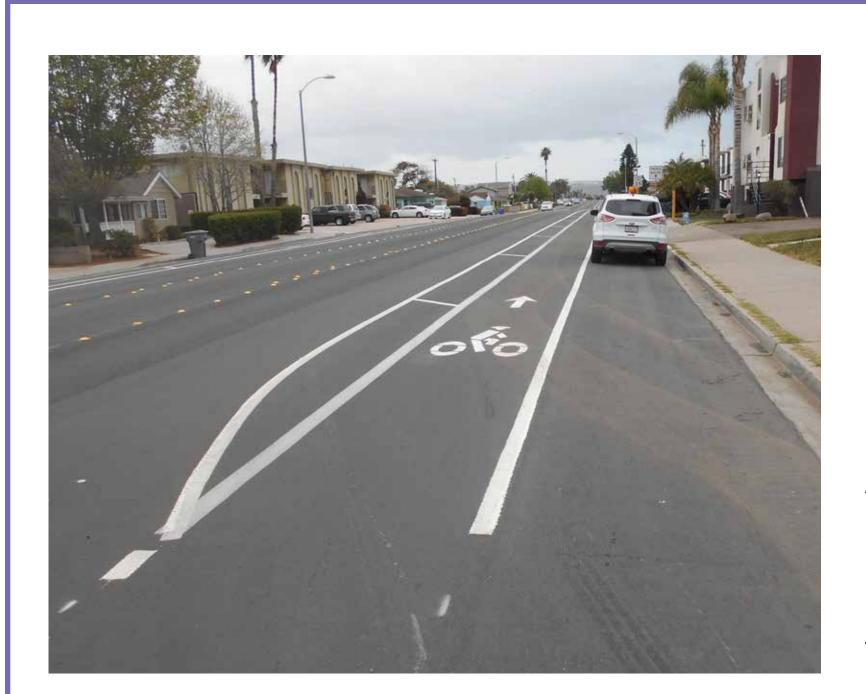
Buffered bike lanes are conventional bike lanes paired with a designated buffer space that helps to further separate people on bikes from the adjacent motor vehicle travel lane and/or parking lane. Buffered bike lanes would be installed on San Diego Avenue (from Noel Street to just east of Hortensia Street) and on Congress Street (from just west of Mason Street to Taylor Street).
