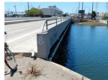
North side of Chollas Creek bridge.
