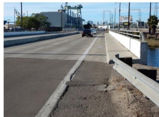
Chollas Creek bridge, looking north.
