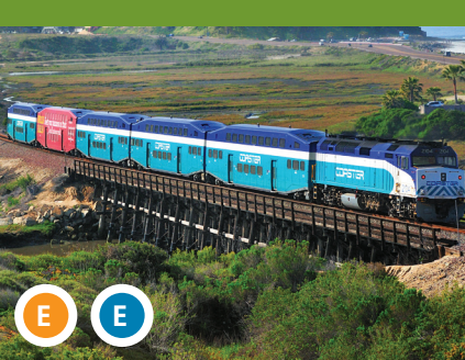
Lagoon Bridge Replacements*
