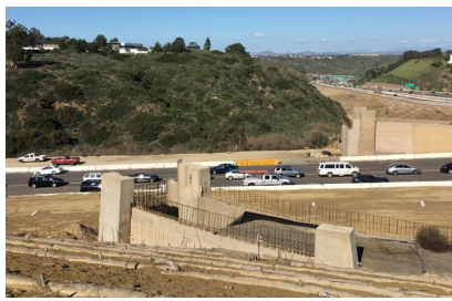
Preliminary construction of the bicycle/pedestrian bridge.
