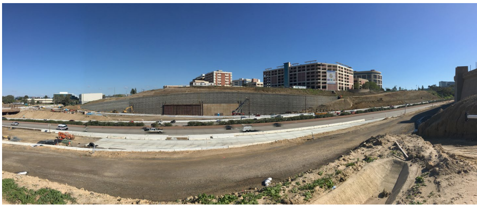
Crews near completion of the retaining wall along northbound I-5.
