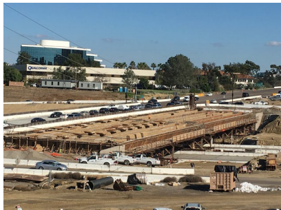
The new Genesee Avenue overpass will accommodate 10 vehicle lanes.
