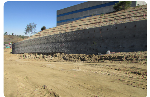
A new retaining wall being built along the northbound on-ramp
