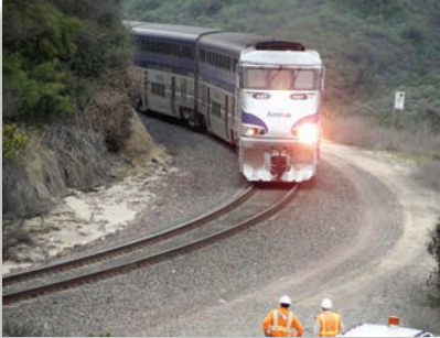
Sorrento to Miramar Double Track Phase II
