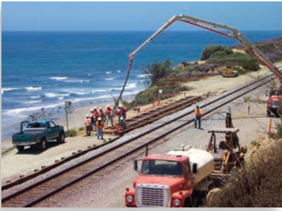
Del Mar bluffs track bed stabilization
