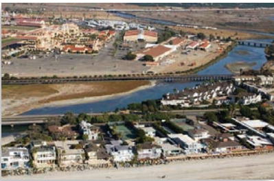
San Dieguito Lagoon bridge replacement
