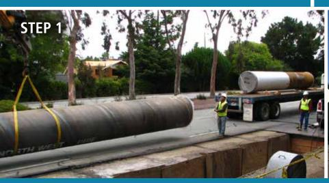
**RELOCATE UTILITIES** Moving overhead and underground utilities out of the way to make room for trolley infrastructure
