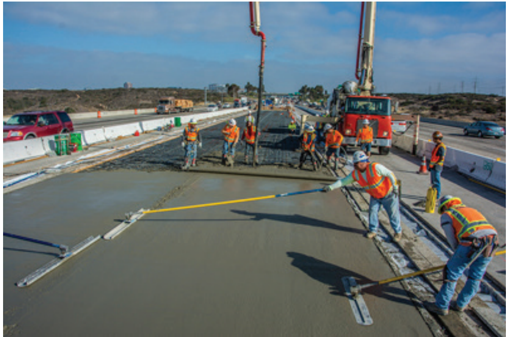
Construction crews pour concrete on bridge deck of Interstate 805 at Rose Canyon.
