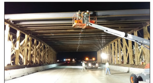
Setting I-beams for the East Palomar Street Bridge.
