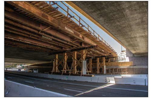
Bridge falsework on I-805 at the Mira Mesa Boulevard undercrossing. Bridge falsework is shown on the left next to the existing northbound off-ramp to Mira Mesa Boulevard.
