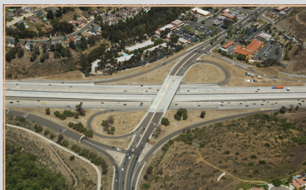
Example of a partial-cloverleaf with loop on ramps—the type planned for the SR 76
