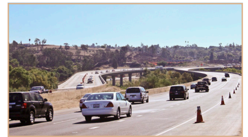
The SR 76 Middle Segment new westbound lanes & improved eastbound lanes
