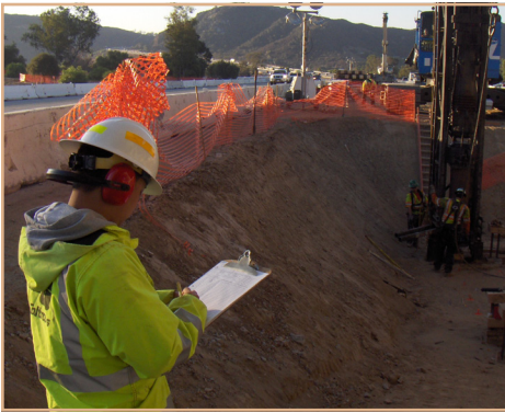
Caltrans Transportation Engineer Victor Yoon inspects the pile-driving work
