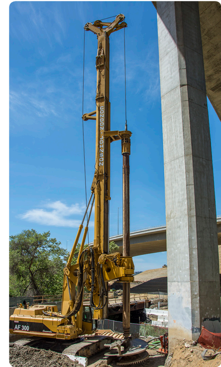
Equipment used for drilling the bridge foundation for I-805, which will be widened along the outside to provide additional lanes.
