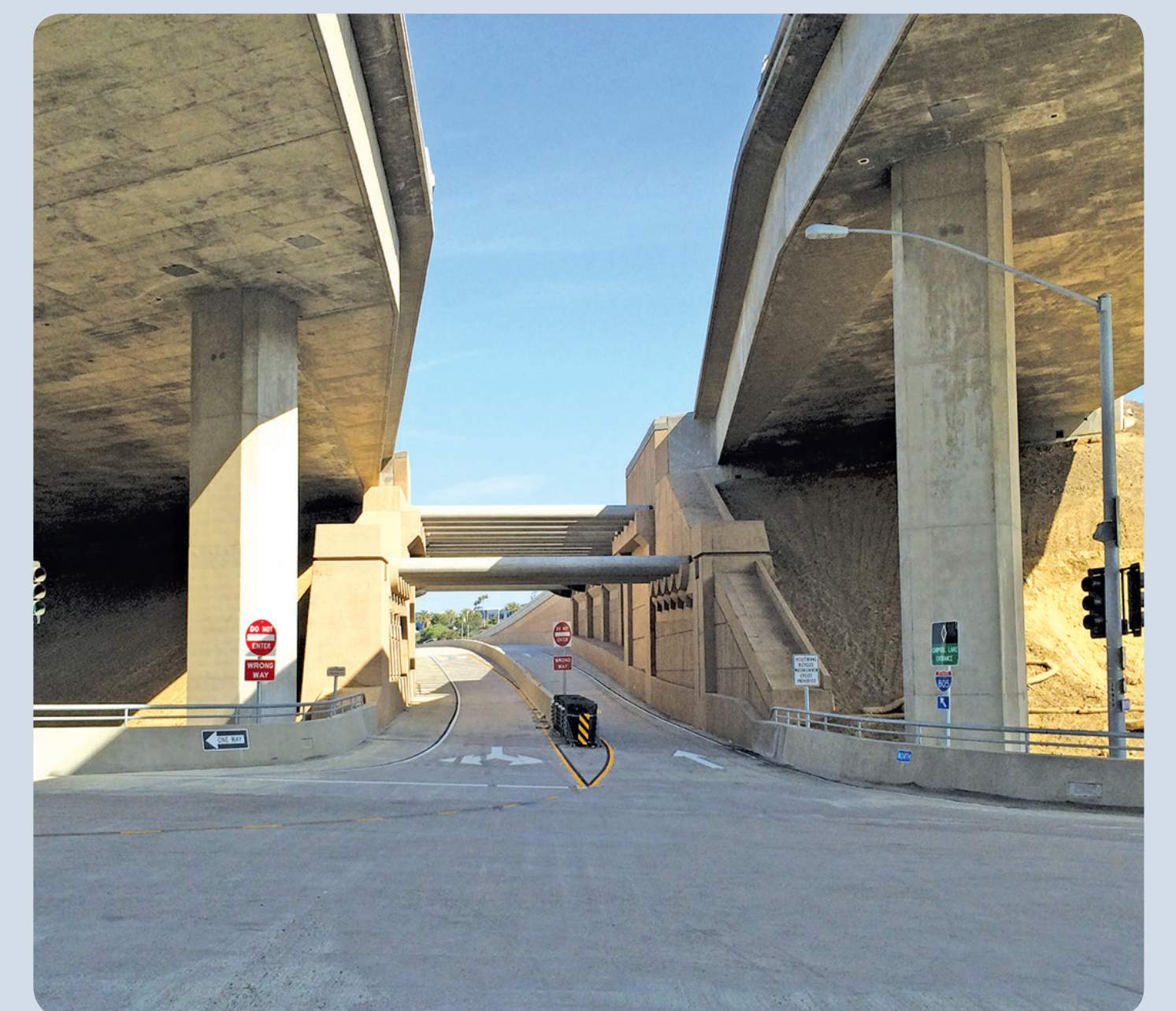
Existing north-facing Direct Access Ramp
