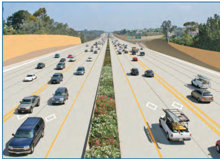
The Locally Preferred Alternative will add two Express Lanes in each direction along I-5, separated by a striped buffer.
