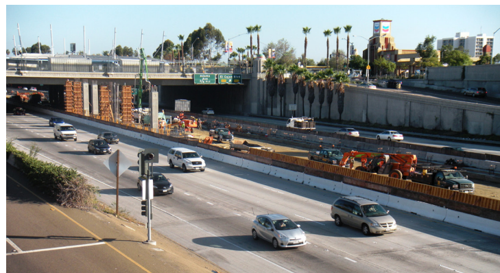
Crews pour concrete columns in preparation for the future pedestrian stairwell south of University Avenue.
