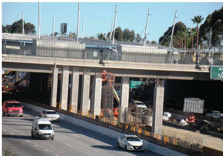
Seven concrete columns have been formed south of University Avenue for the future pedestrian stairwell.
