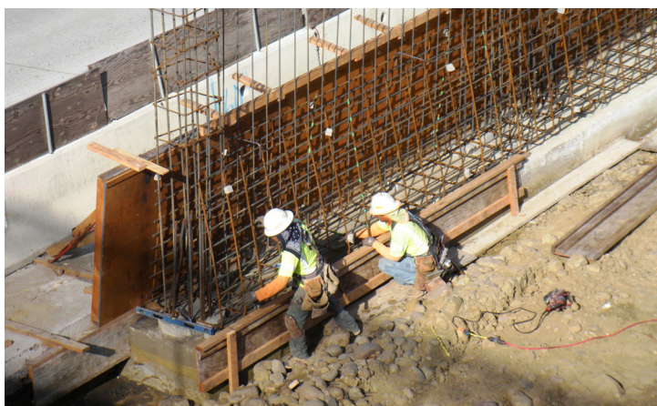
Construction crews form transit station walls in the SR 15 median south of University Avenue.
