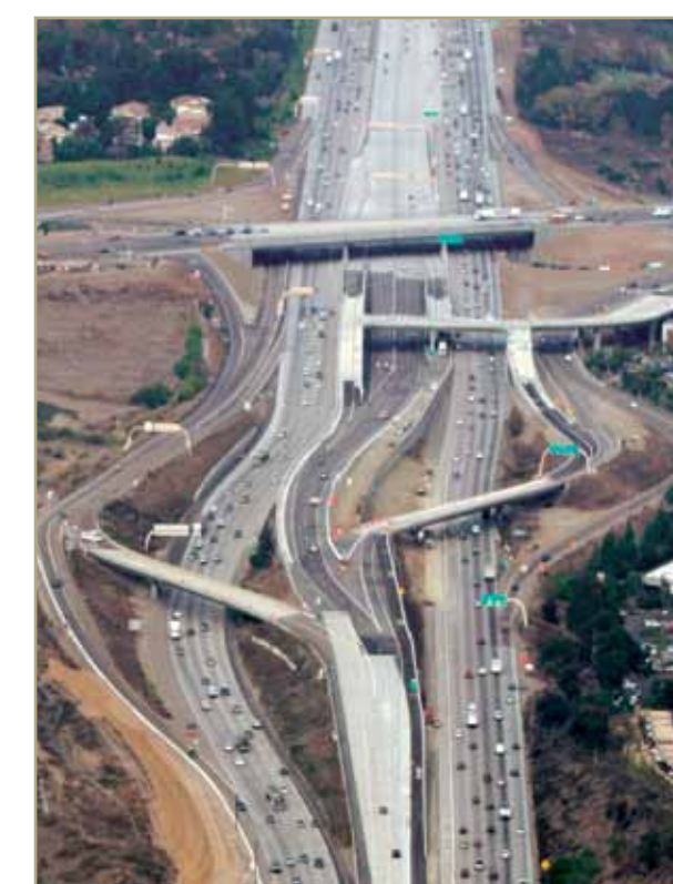
Construction of the DAR at the Sabre Springs/Peñasquitos Transit Station: aerial view looking north.
