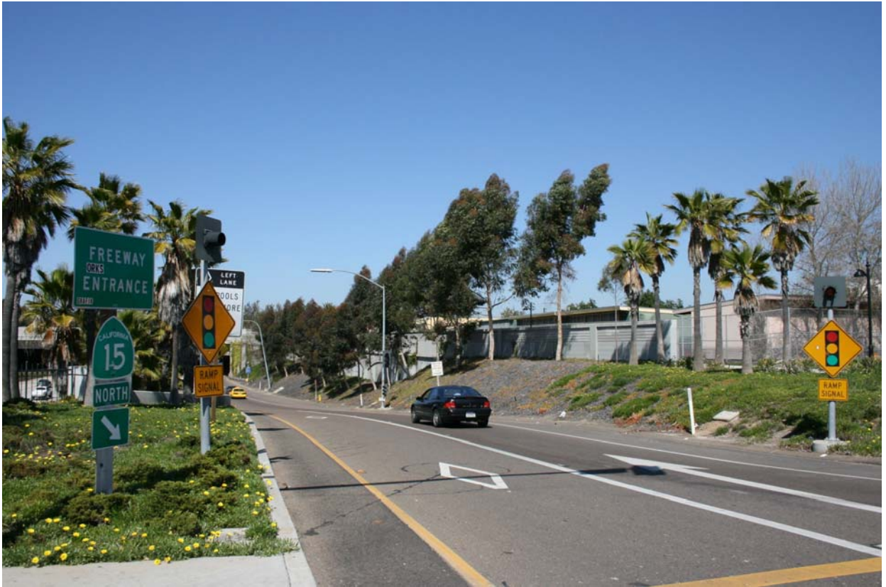
Existing Conditions: View looking north at SR-15 Northbound On-Ramp near University Avenue
