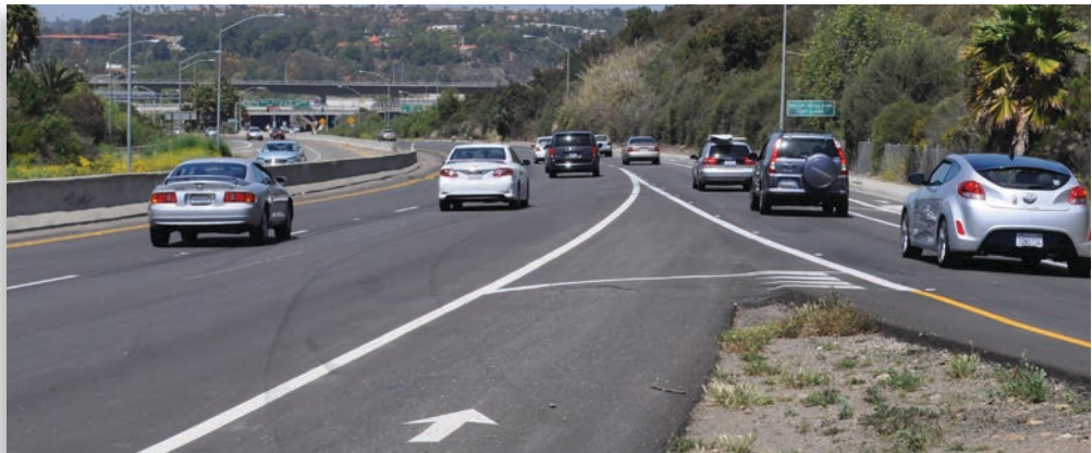
Fairmount Avenue - Looking north on Fairmount Avenue where the westbound Montezuma Road ramp merges onto northbound Fairmount Avenue, showing high-speed traffic conflicts as vehicles travel through the path of bike riders.
