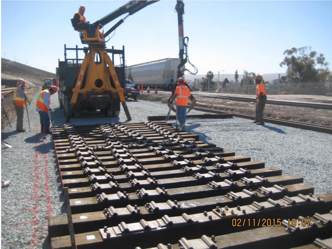
**Photo 4 – Crossover Construction in Progress**
