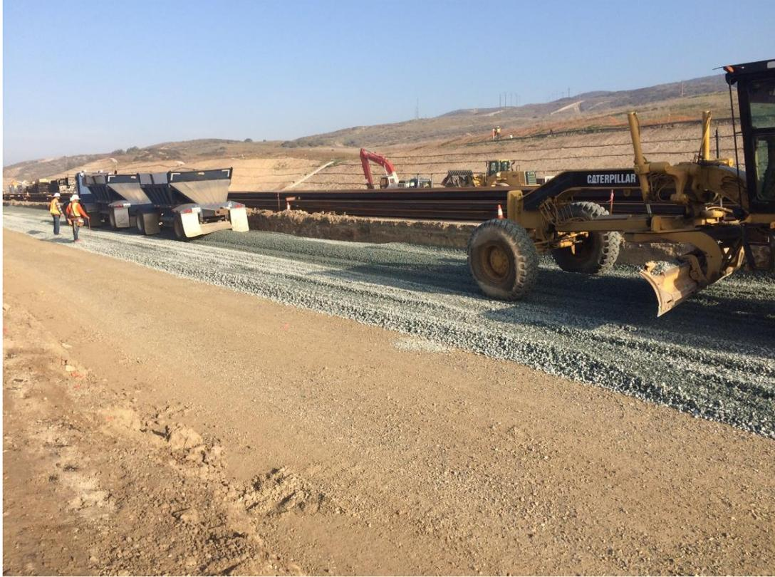
**Photo 2 – Track Ballast Installation in Progress**
